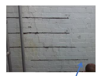
Wall cracking repaired using a proprietary product (Helifix)
